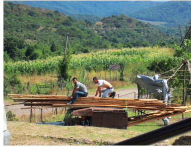
The wood used for the construction of One Caucasus Town in 2014 and 2015 were transported and stored in Tserakvi school.
